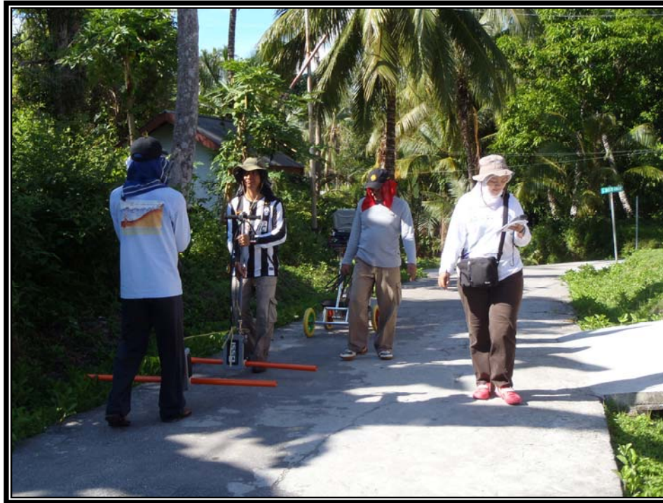
Figure 3. Operating of Ground Penetrating Radar with 3200 MLF antenna
