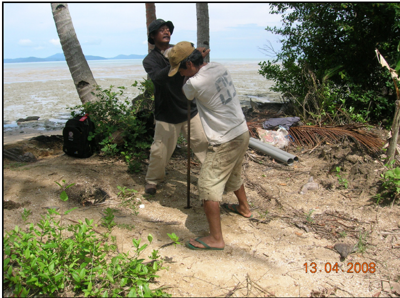
Figure 5 Location of hand auger drilling BT 18 at the Sawah Bay
